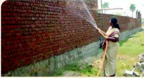
Curing the brick Walls
