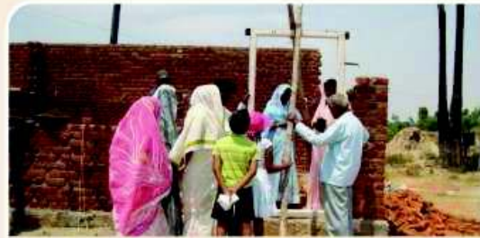
Fixing the Door Post
